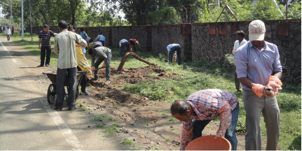
Shramdaan for pit-filling
